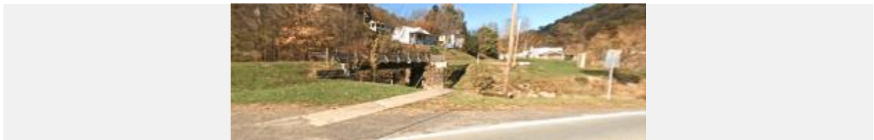
Modern view of the second burned span at Church’s Fork. Today the B&O track has been converted to a popular rail trail (Google Streetview)
